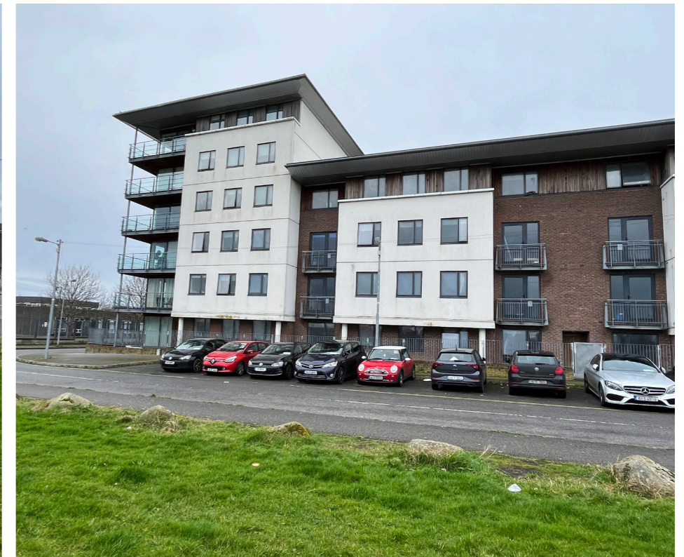
Fig: 12. Site photo looking West, towards Gateway Student Village
